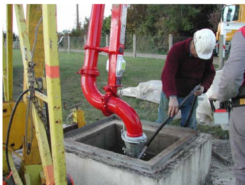
Injection de ciment
